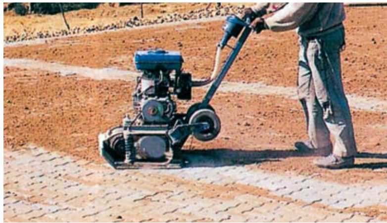
Vibrating the jointing sand into the joints
