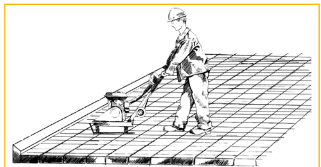
Figure 16: Vibrating the blocks into the bedding sand layer
