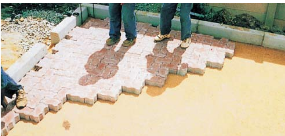
Commencement of laying establishing a diagonal face
