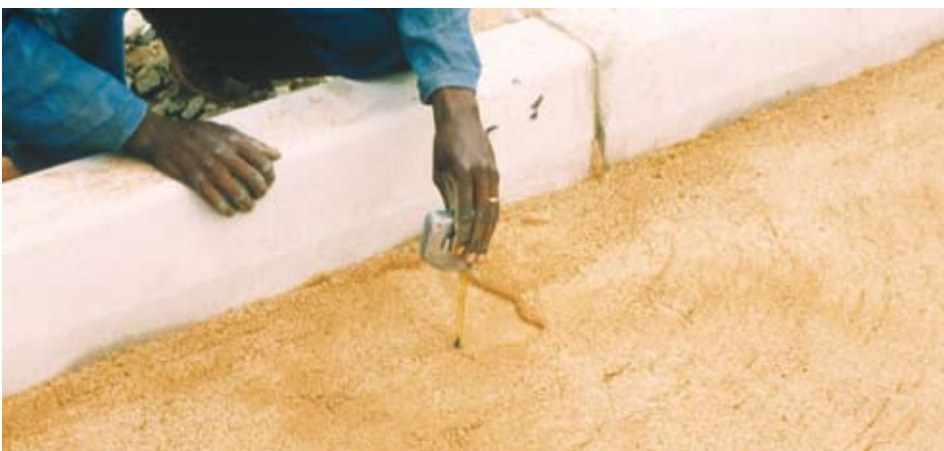
Edge restraints installed before laying commences
