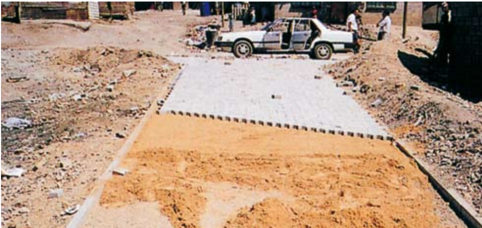
Typical site layout/ construction sequence
